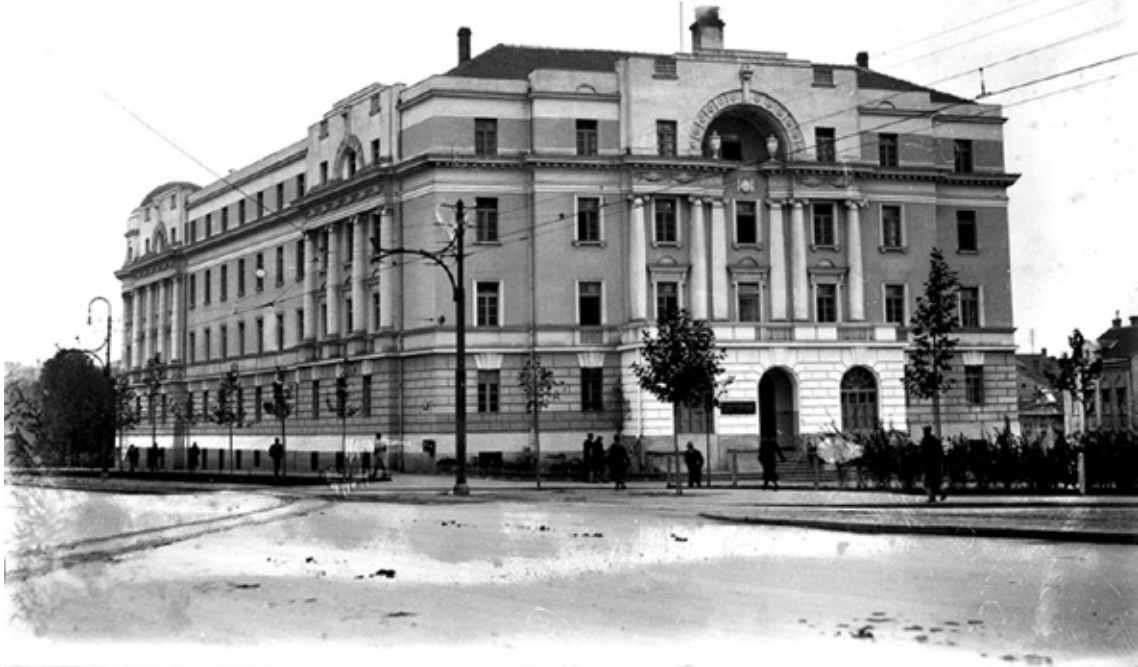
Fig. 6. Students' Dormitory of King Alexander the First (1926–1928), architect Grigory Pavlovich Kovalyevsky
