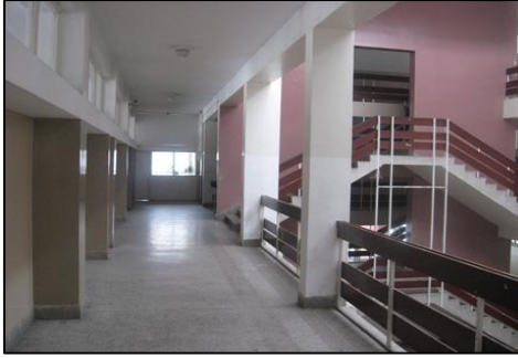
Figure 1. Interior part of the Electrotechnical school „Nikola Tesla” in Niš (figure source: Jevtić, B. R., Ničković, T. J., The determination of fire propagation by simulation ).
