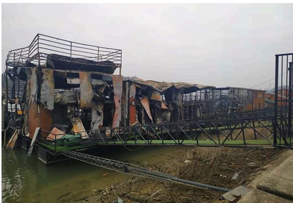
Picture 3. This photo shows several problems: Illegal floating night-clubs; illegal electric and water installations that brought to a major fire; a view over the river that is completely blocked; polluted water by litter thrown from these floating objects. January 2020. Source: Za nas kej.
